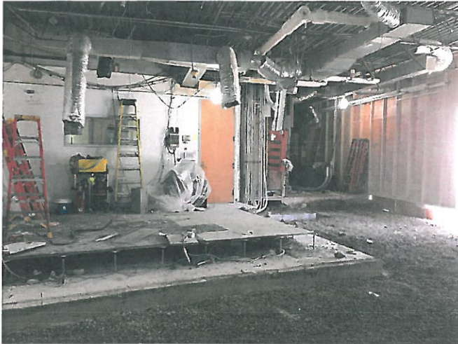
911 Center Floor Prepared
