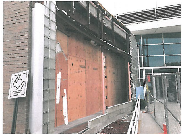
Building Department Wall Being Taken Down
