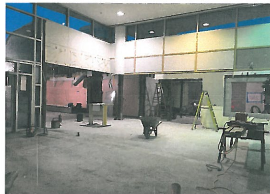
Lobby Work Area
